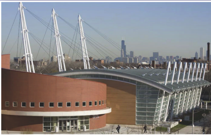
2004 EAE National Winner – 310 tons of beams bent including reverse curves for the Gerald Ratner Athletics Center. Chicago, IL.
