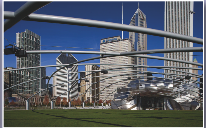
2005 EAE Merit Award – 570 tons of 12, 14, 16, 18, and 20 inch pipe curved for the Jay Pritzker Pavilion. Chicago, IL.
