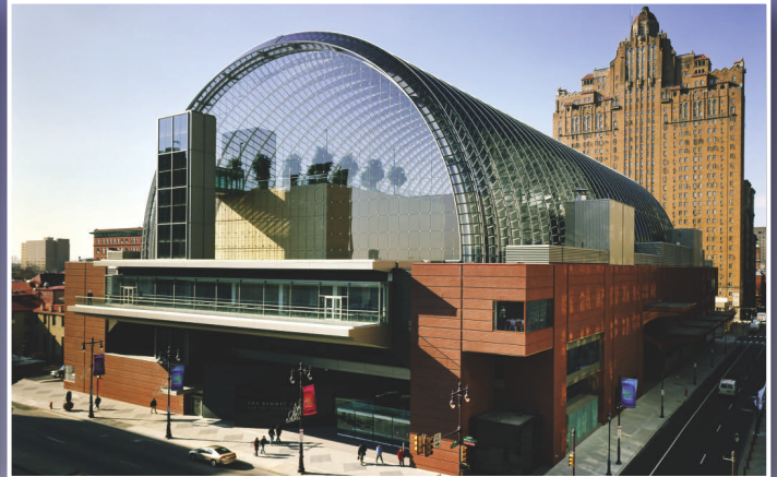
2003 IDEAS 2 National Winner – 300 tons of 5 inch square tubing curved 45° off-axis for the Kimmel Center. Philadelphia, PA.
